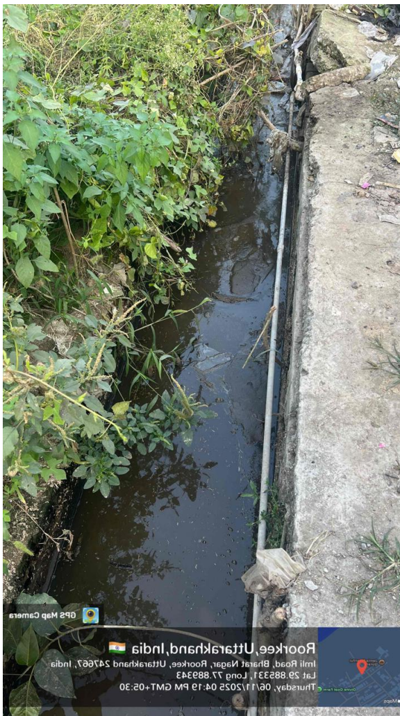
Figure 12: Imli Road, Bharat Nagar Drain, Roorkee, UK
