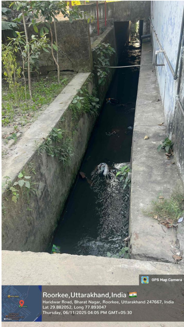
Figure 9: Bharat Nagar Drain, Roorkee, UK
